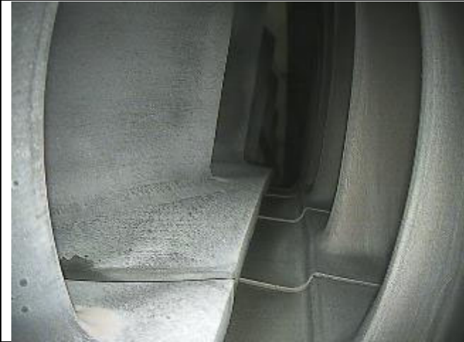
HPTN2 T/E and Inner Platform
