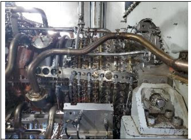
External View HPC VSV Right Side
