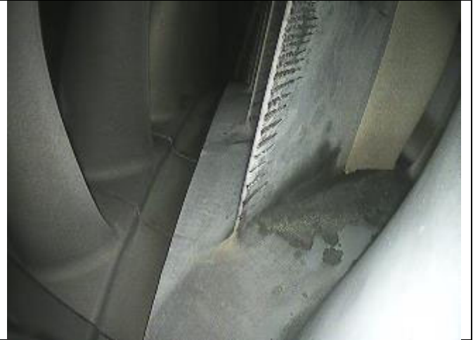
HPTN2 T/E and Inner Platform.
