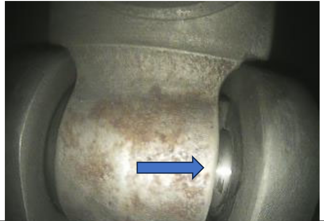
VBV Inspection / Door Hinge Bushings Broken/Missing
